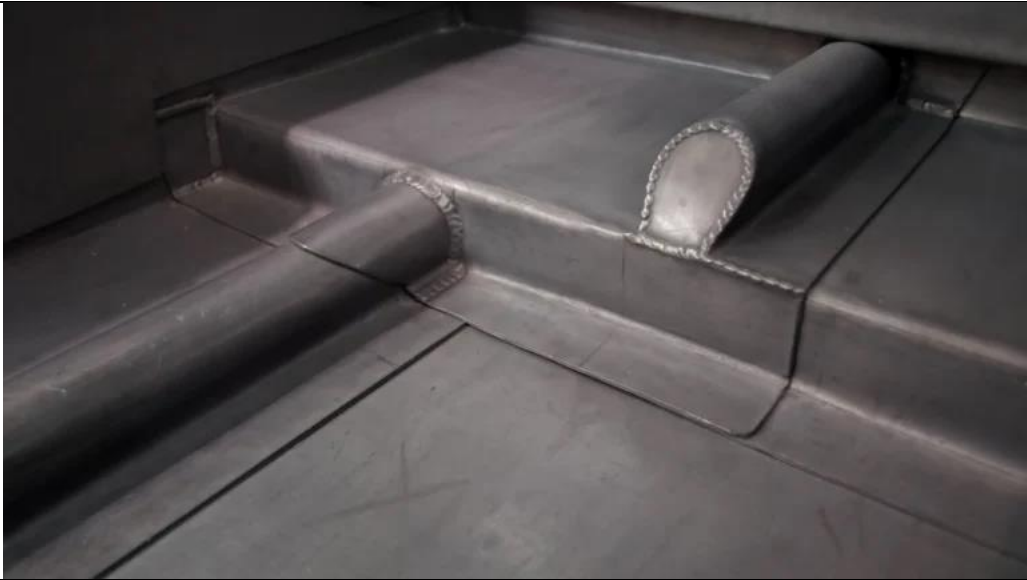
Image 2: lead welding finish
