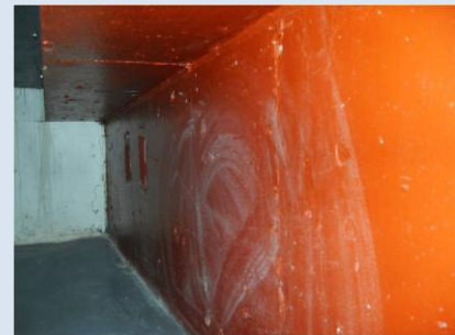
Low level areas beneath plant and equipment
