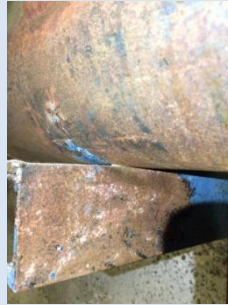
Beneath pipes especially where brackets or supports are present
