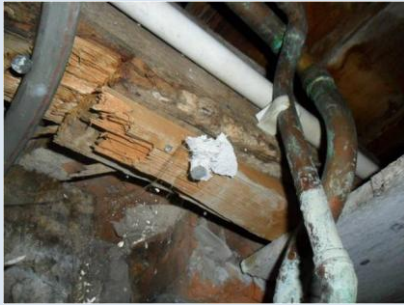
Timber batons where AIB has been attached
