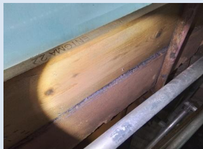
Scaffolding boards and gaps between them
