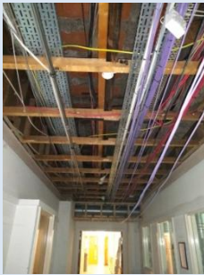
Ceiling supports or walls where ceilings were attached
