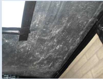
Polythene sheeting including the airlock and baglock
