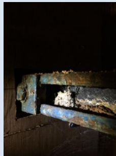
Within cavities and supporting brackets
